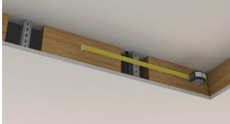
Measure structural mounting points in the ceiling where the LUXCANVAS will be secured to.
