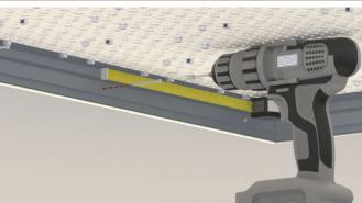
Based on the locations of the structural points, pre-drill holes in the side wall of the LUXCANVAS frame, making sure to avoid any wiring or electrical components.
