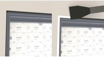
Apply mudding to seal the gaps between the aluminum frame and the ceiling structure.
