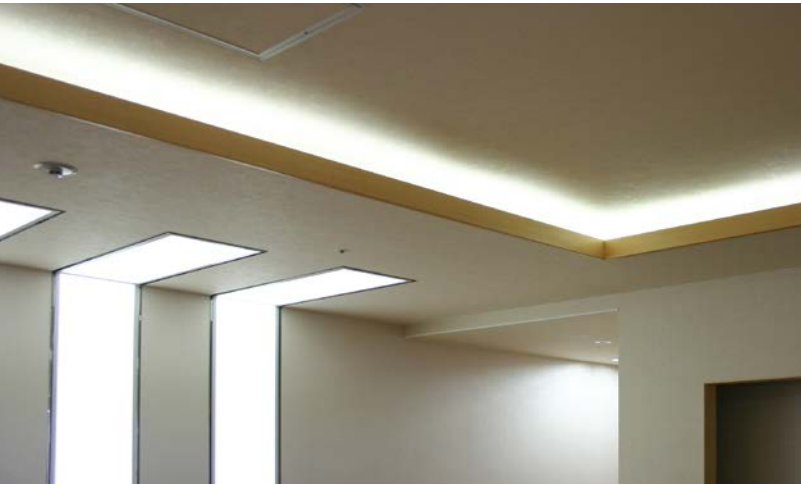
INTERIOR COVE LIGHTING
